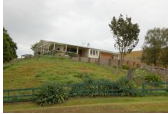
Photo 14: Adjacent house to view in photo 13.
